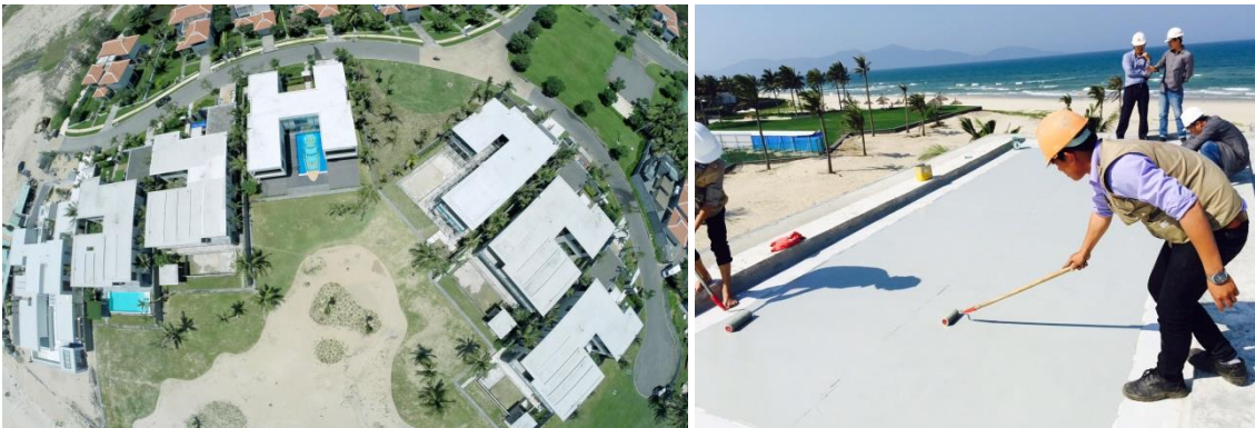
Picture: Sikalastic 632 was applied at Ocean Villa project
