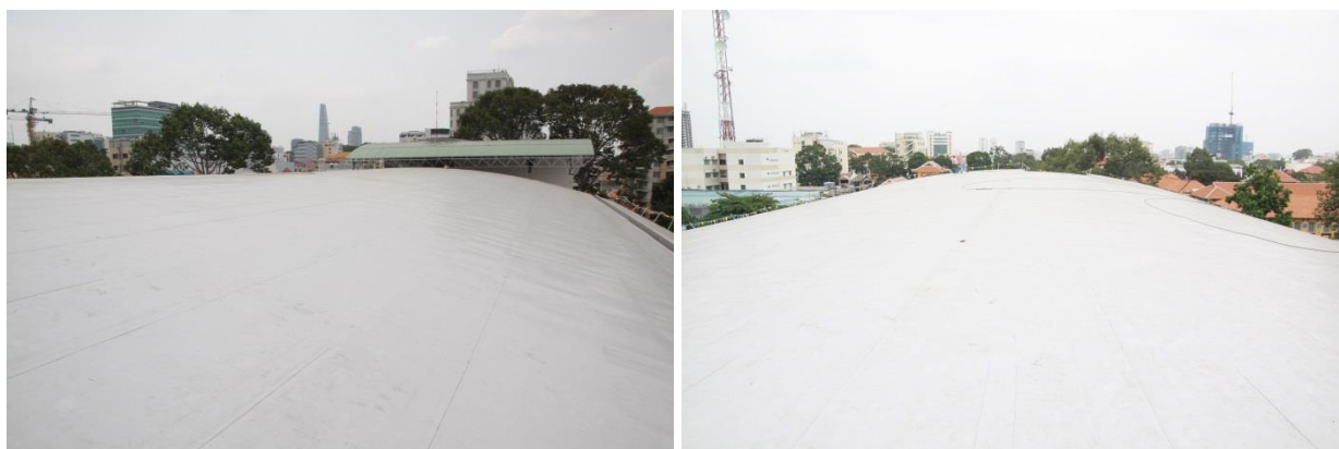
Picture: Sarnafil® S327-15EL was applied at Ho Xuan Huong sport Center project
