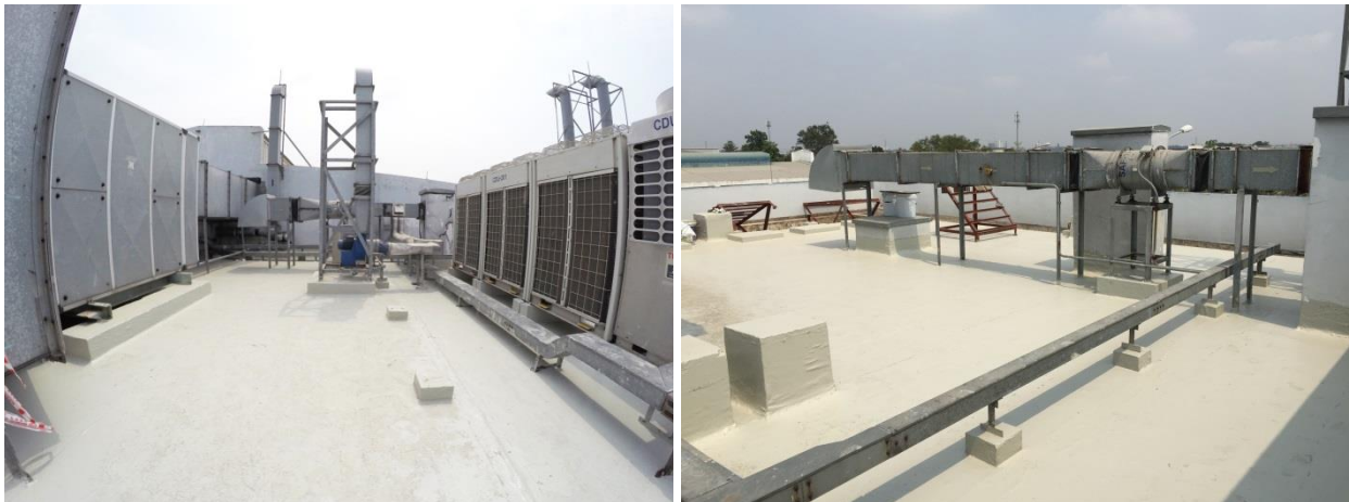
Picture: Sikalastic 632 was applied at Akzo Nobel factory project
