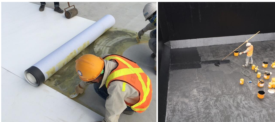
Picture: Sarnafil® G-410-12L Felt and Sikafloor Epocem 81 were applied at Nestle factory projects
