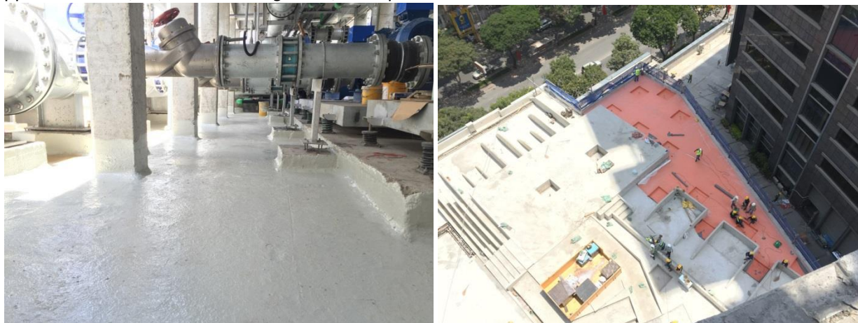
Picture: Sikalastic 632 and Sarnafil G-476 were applied at Sai Gon Center Phase 2&3 project
